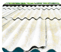
Asbestos sheets
